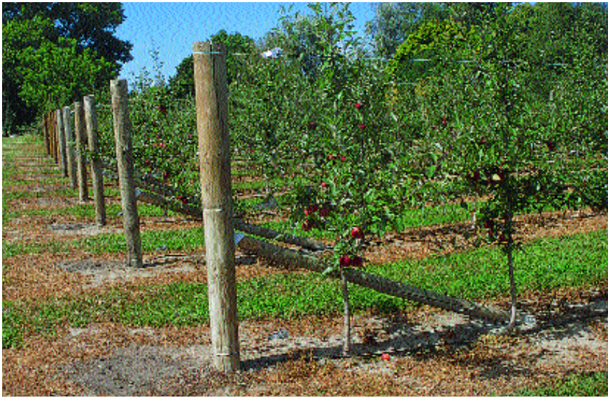
This unique end-brace structure eliminates the need for an anchor outside the trellis system by using wired "push-pull" forces within the wooden support.
